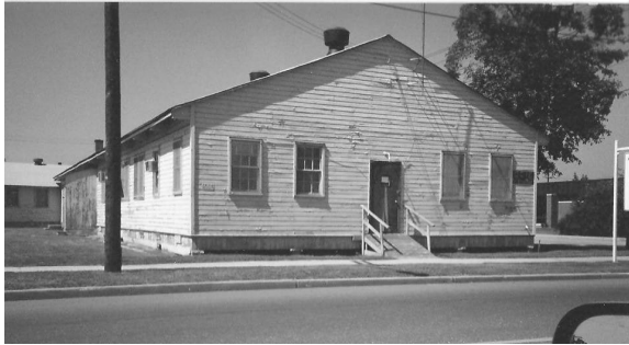
Typical Army Office Building at Camp Croft
