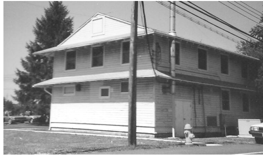
Typical Barracks at Camp Croft
